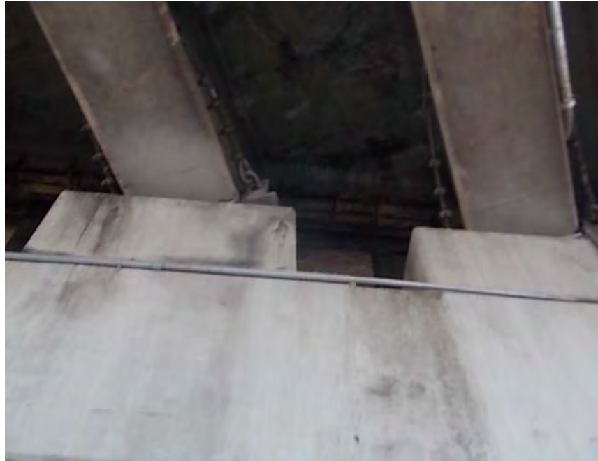
DIAPHRAGMS SPAN # 2 SPALL TO STEEL AREAS
