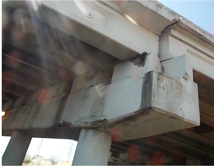
BENT # 1 REAR RISER BLOCKS SPALL TO STEEL
