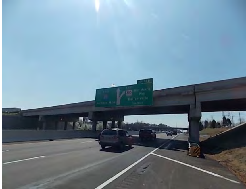
SIGN AT SPAN # 2 LEFT SIDE OF BRIDGE
