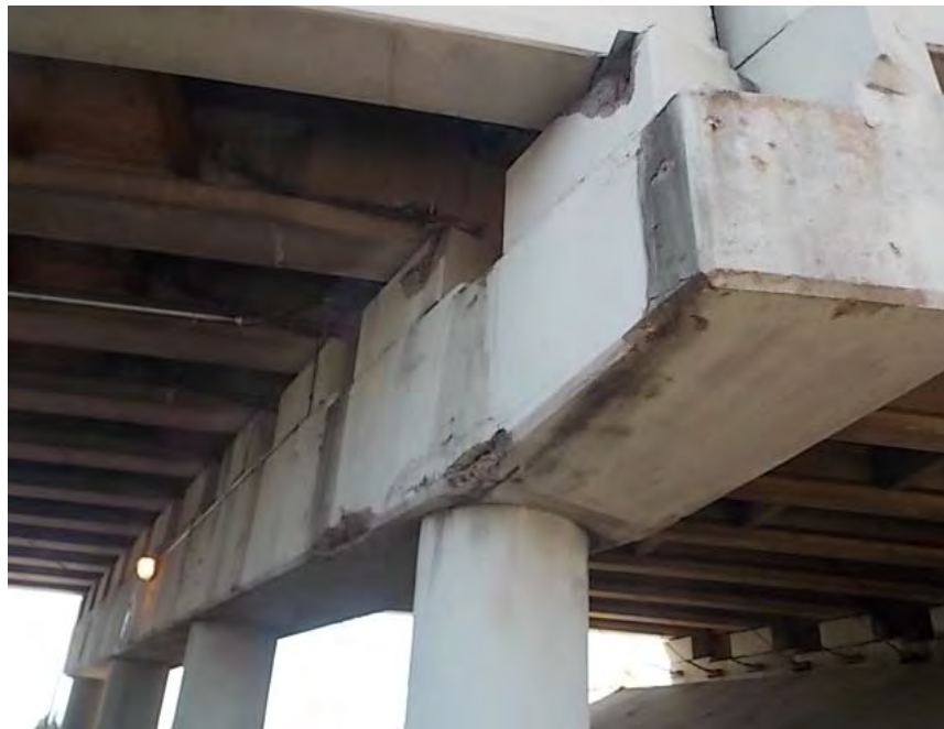
BENT # 1 REAR RISER BLOCKS SPALL TO STEEL
