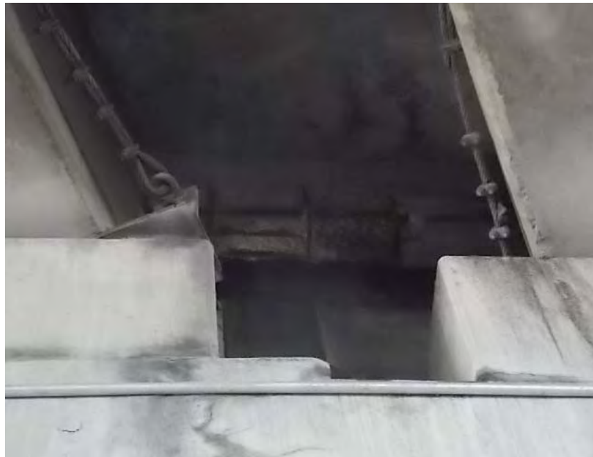
DIAPHRAGMS SPAN # 2 SPALL TO STEEL AREAS
